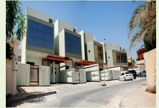
33 Units 2-Storey Villa in Mahooz
