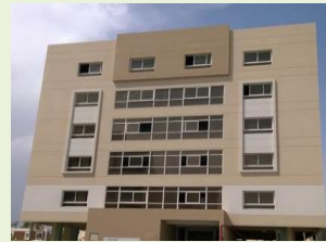
7-Storey Building in Juffair
